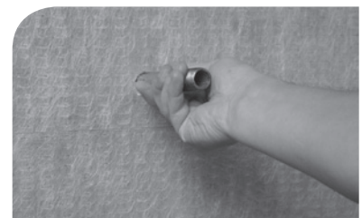
Replace plumbing pipe into backboard ensuring to use proper plumbing practices.
