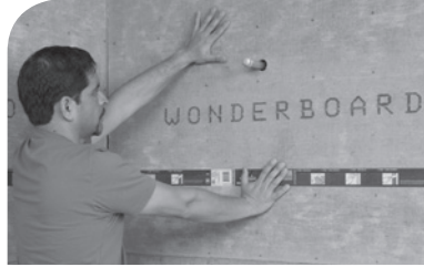
Install 1/2" (13 mm) cement backboard for wall installation. Cut open areas to support plumbing fixtures.
