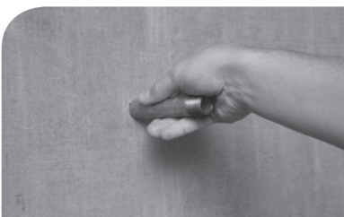
Remove plumbing protrusion.
